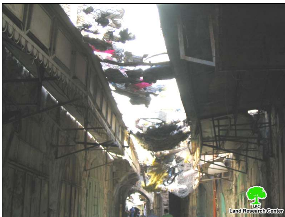
One of the alleyways in Al Qasab Suq provided with metal netting
